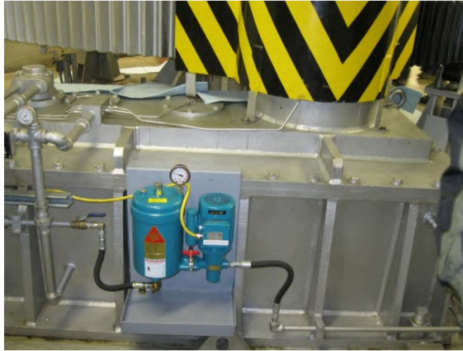
Figure 6-4. Kidney Filter for a Gearbox.
