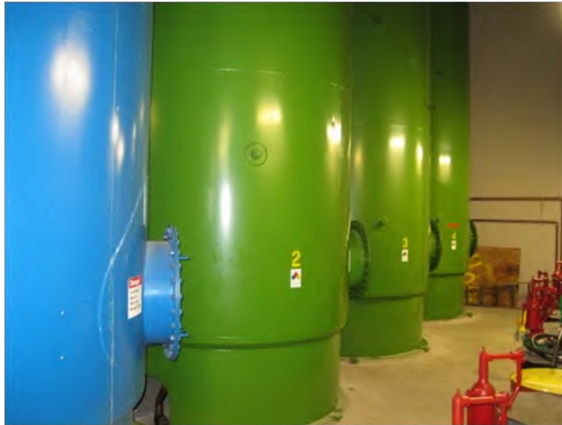
Figure 8-1. Hydroelectric Plant Turbine Oil Storage Tanks.
